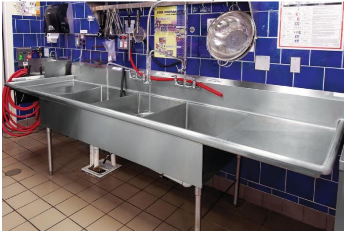
Three-Compartment Sink w/ Sanitary Sink
