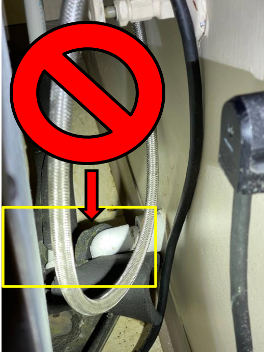
Ice Machine installed with No Air Gap, Directly connected to Sanitary Sewer System.
