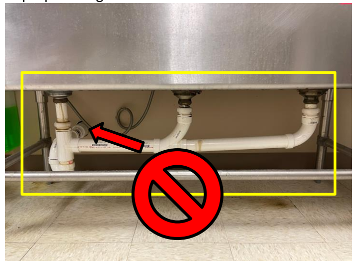
Three-Compartment Sink with No Air Gap, Directly connected to Sanitary Sewer System.
