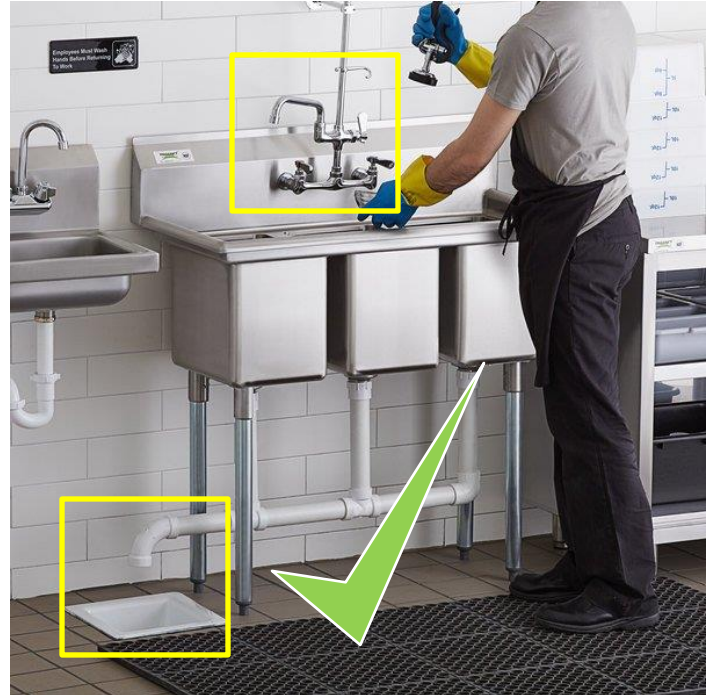
Required Two Air Gap Design Into Floor Sink.
